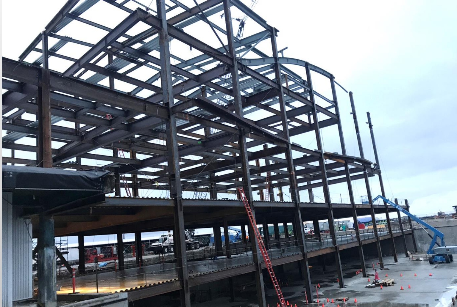
Phase 1 from NSAT Roof 1/3/18
