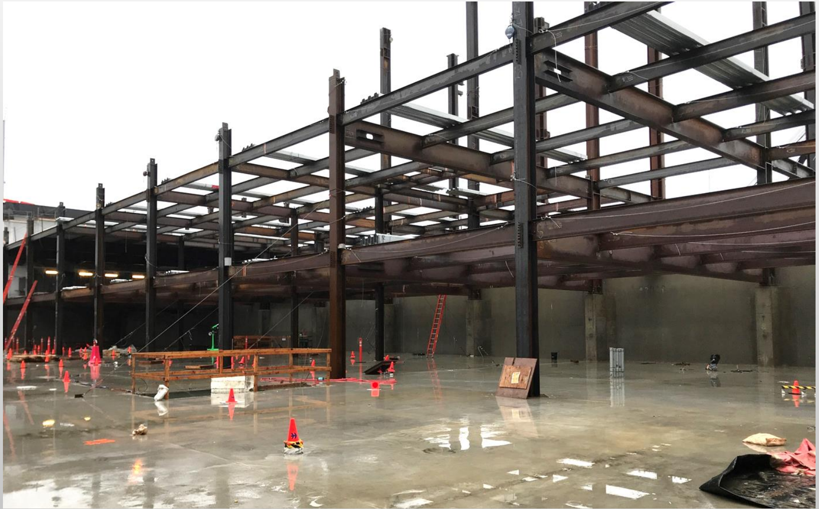
Phase 1 Basement View 1/3/18
