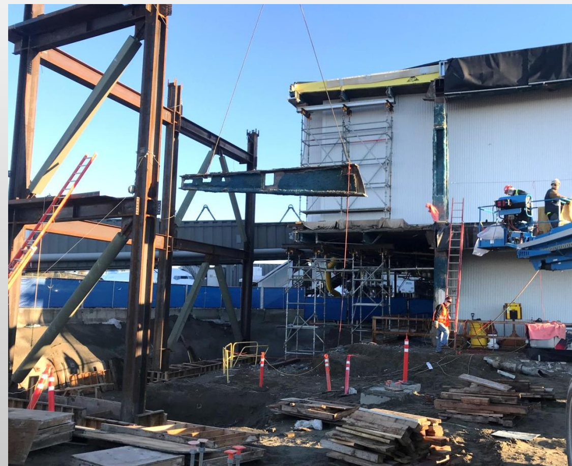
New Steel installation progress 12/4/17
